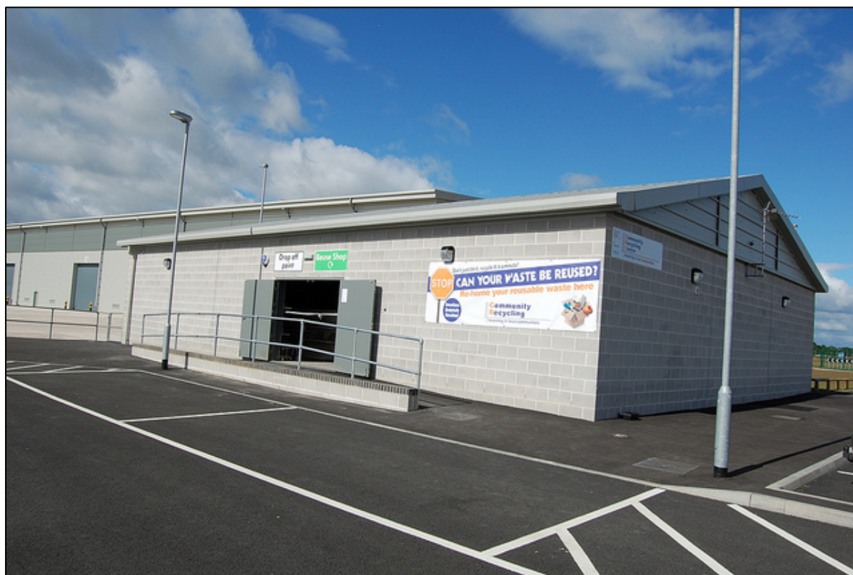
Photo 6 Lower House Farm re-use shop
